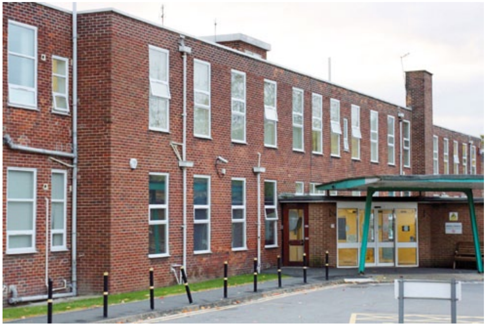
The Guisborough Hospital site
