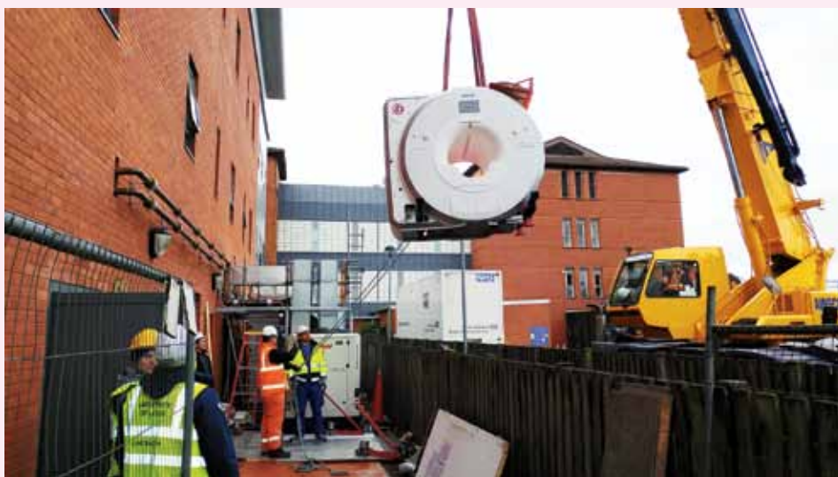
The scanner is lifted into the Friarage Hospital (Picture courtesy of Interserve)
